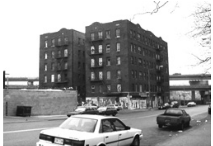
Fig. 3. Casa del Sol/FUTURE CITY as it exists today. The photograph is taken looking south towards the Bruckner Expressway.
